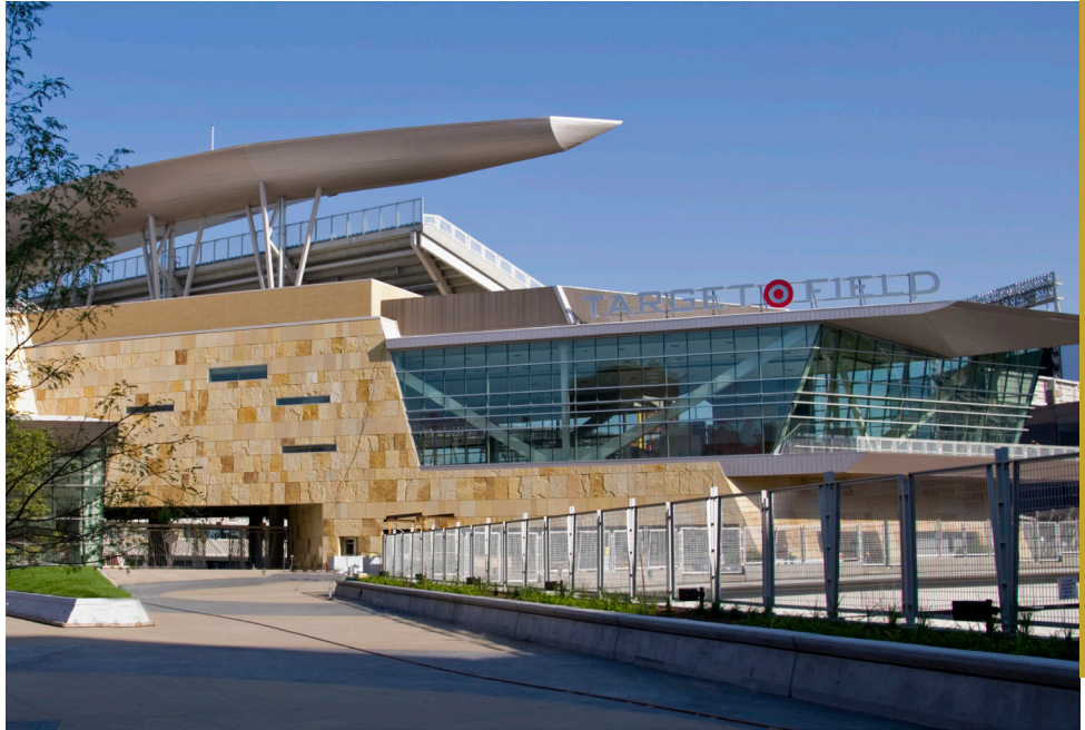
Target Field - Minneapolis, Minnesota, United States Architect: Populous Architects | Photo Credit: Kevin Wood Photography
